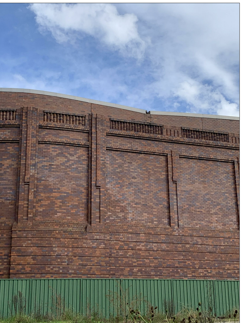
VIEW FROM SITE TO SYDNEY WATER RESERVOIR
