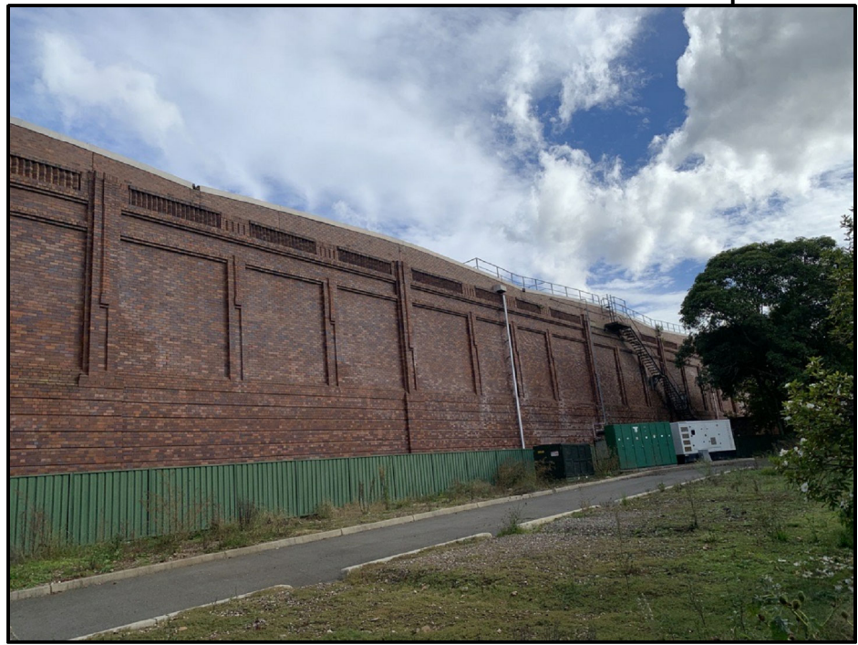
SYDNEY WATER RESERVOIR BRICK WALL
